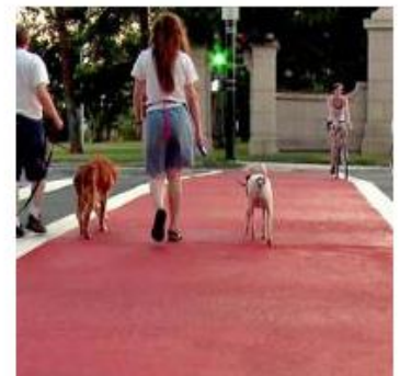
DECORATIVE STREET SURFACE Decorative street surfaces include contrasting materials such as pavers or paint to help define pedestrian crossings and activity spaces. The contrast in texture or color helps define areas that are safe for pedestrians, while alerting motorists to take extra caution when approaching.
